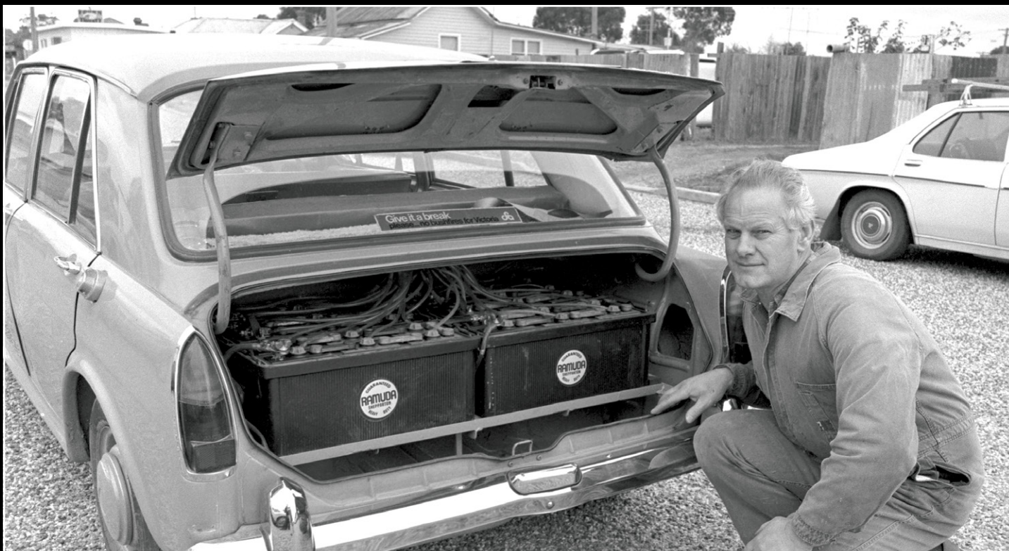
Mr Neil Harris, from Seymour in Victoria, in 1980 with his 1967 Morris 1100 sedan that he converted to an electric vehicle in 1978. He chose the Morris to convert because of its compact size and it being front-wheel-drive. NAA barcode 11412453
