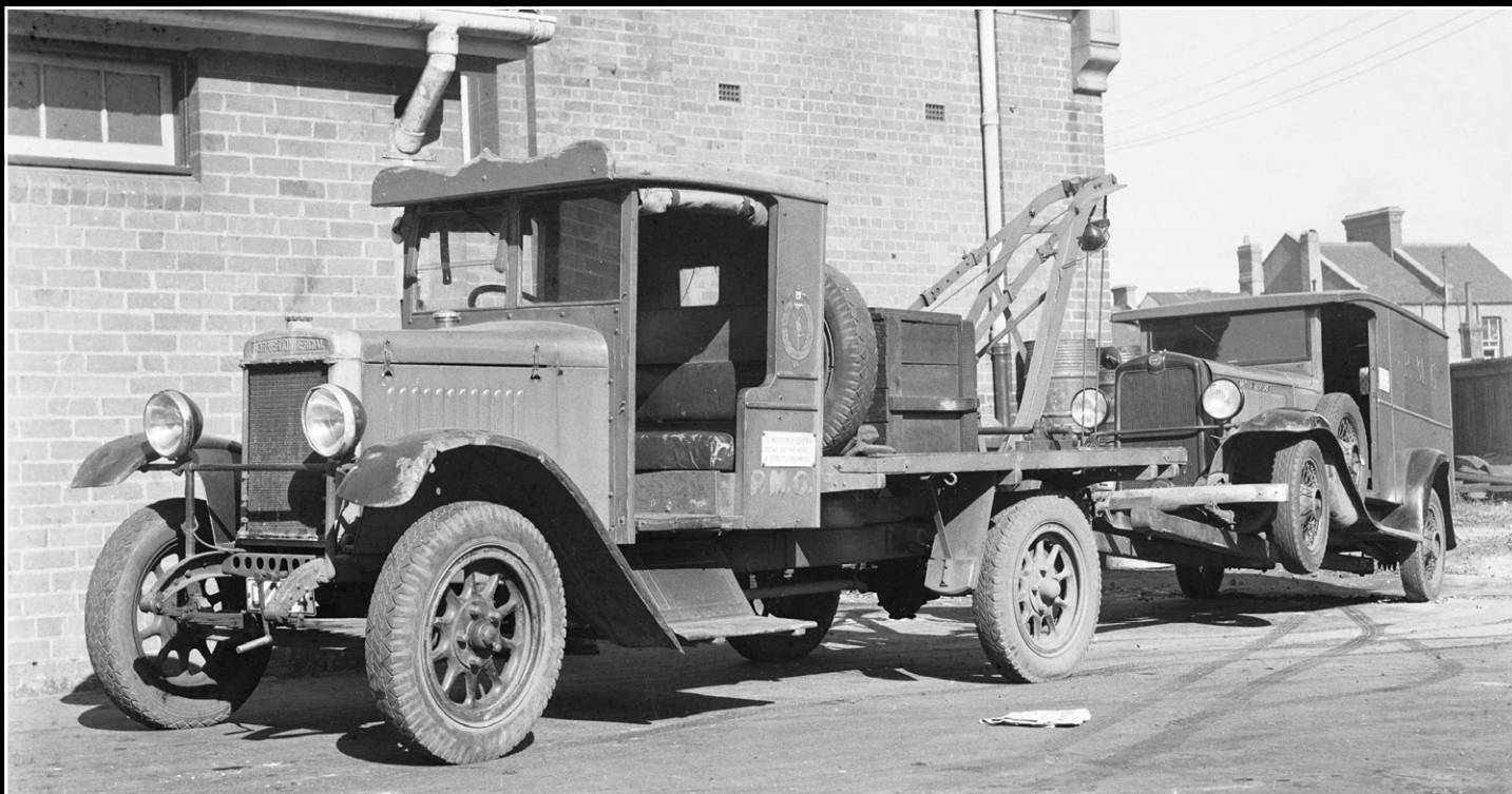
Back in 1939 when this photograph was taken, the Postmaster-General's Department was responsible for all postal and telecommunications services in Australia. Here we have a 1927 Morris Commercial, a little the worse for wear, adapted as a breakdown vehicle, with a British Bedford van in tow. NAA C4078_N1478A barcode 1647655
